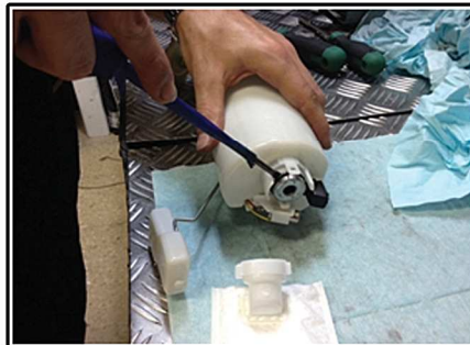
2. Remove the one way valve
